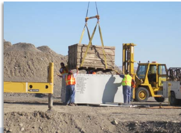
3A Trench 17 Boxes 4-11 Removal and Over-packing
