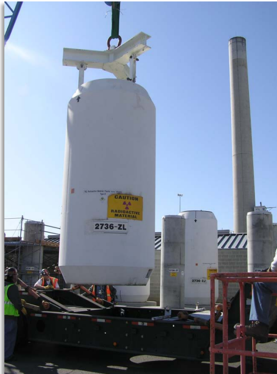
Setting the Interim Storage Container on to the transporter
