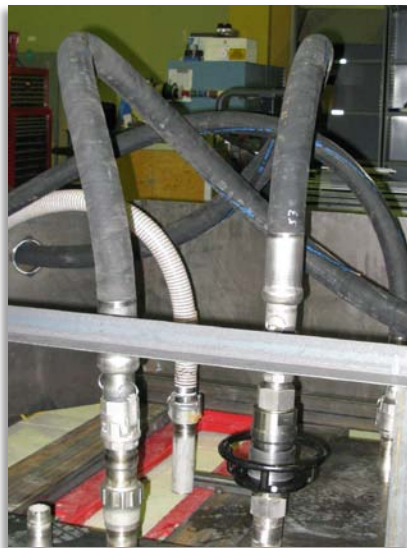
Sludge Transfer Storage Container Hose Connection Test Setup
