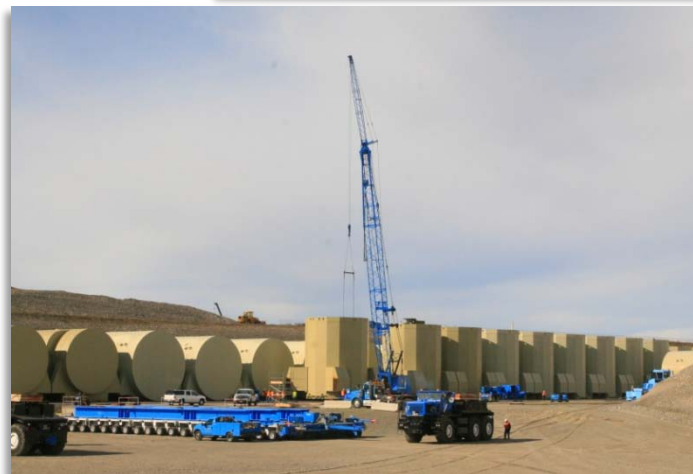
EX-USS-South Carolina RC at Trench 94
