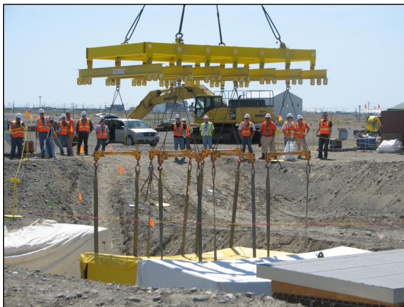
MSA Crane & Rigging assists CHPRC with lift of FRP waste box.
