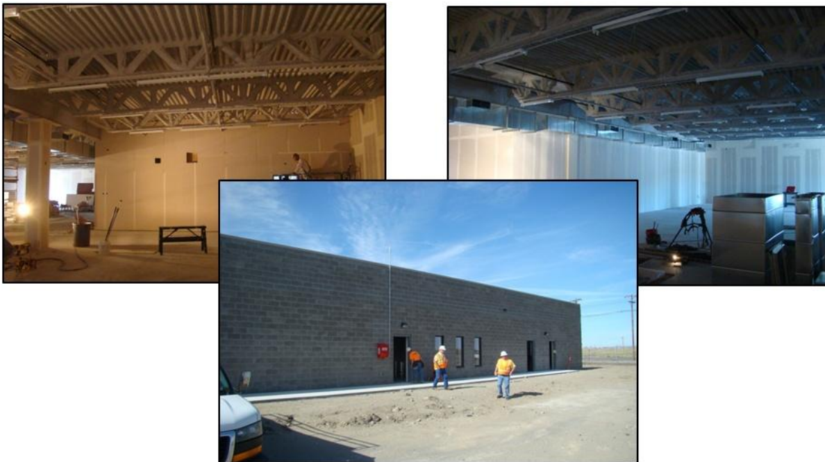
Construction progressing on the new Records Storage Facility
