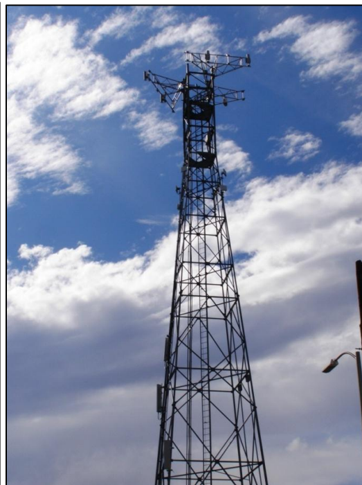
200West Communications Tower
