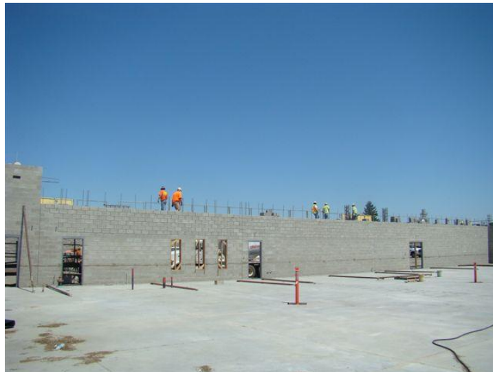
Construction of the new 3212 Records Storage Facility in process
