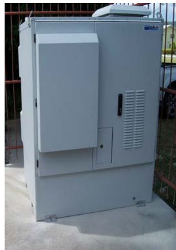
Figure 15: IdaTech PEM Back-up Unit Photo courtesy of IdaTech LLC, NREL/PIX 19192.
