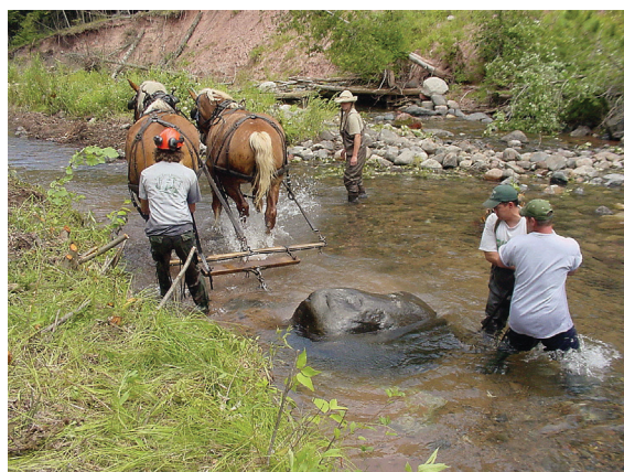
To minimize impact to riparian and aquatic habitat, stream restoration techniques can include use of draft horses to place rock structures. (Photo: USFWS)
