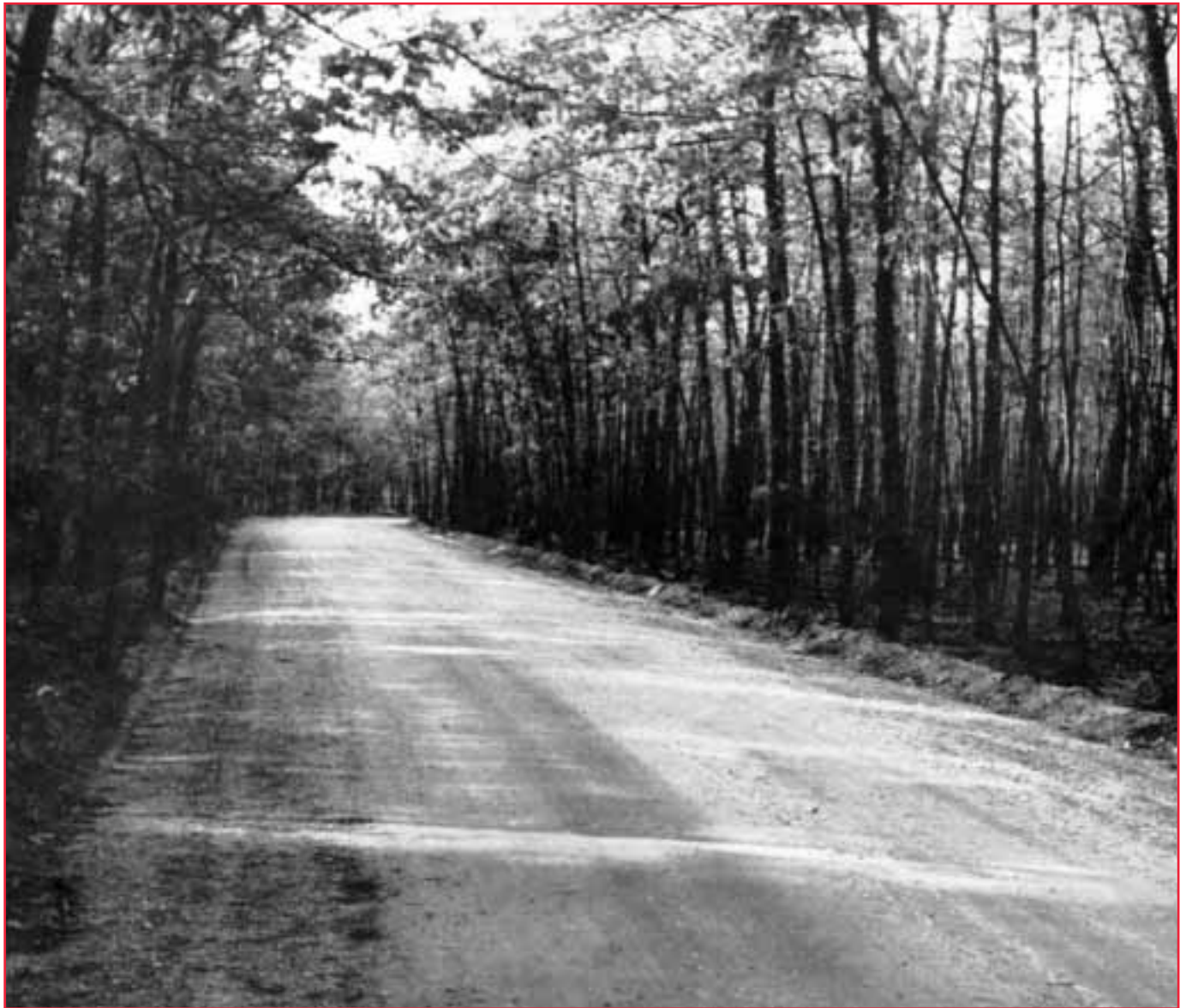
Figure 2 —The stands on both sides of this road had been prescribe-burned in the winter of 1962–63. A good burn had been obtained on the left side, and here the fire of April 20, 1963, burned only a few scattered patches. On the right side, only the top litter had been burned by the winter fire, and much damage was done in April.
