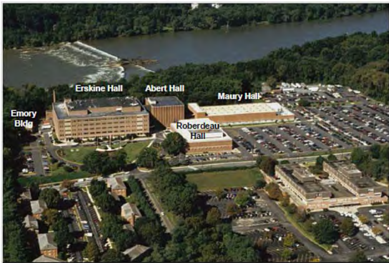
Figure 3: Birdseye view of the existing condition of the installation, looking west (the installation fronts Sangamore Road, which runs through the center of the photograph).
