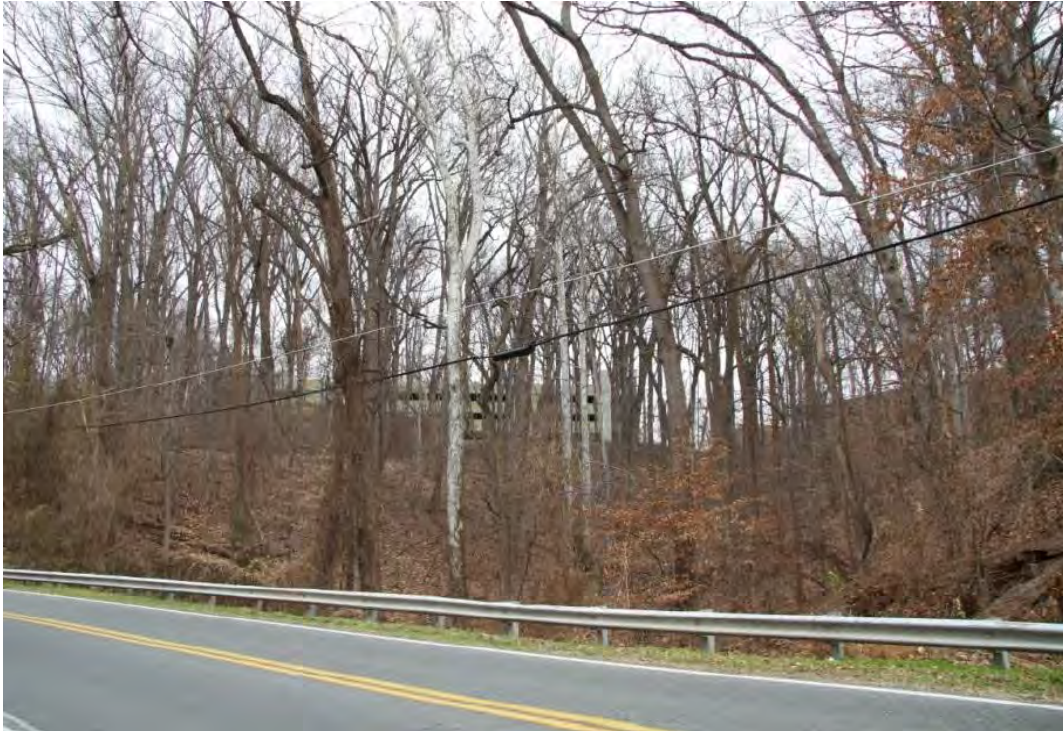
Figure 20: Illustrated view of proposed garage from MacArthur Boulevard; omitted from this view is the proposed screen of evergreen trees and the proposed green screen on the side of the garage.
