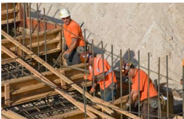
NSLS-II construction site, July 2009
