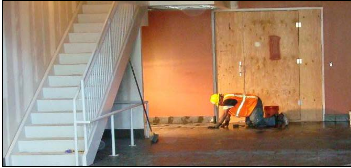
Figure 5. Hand work on the flooring installation near a doorway in pentant 1.
