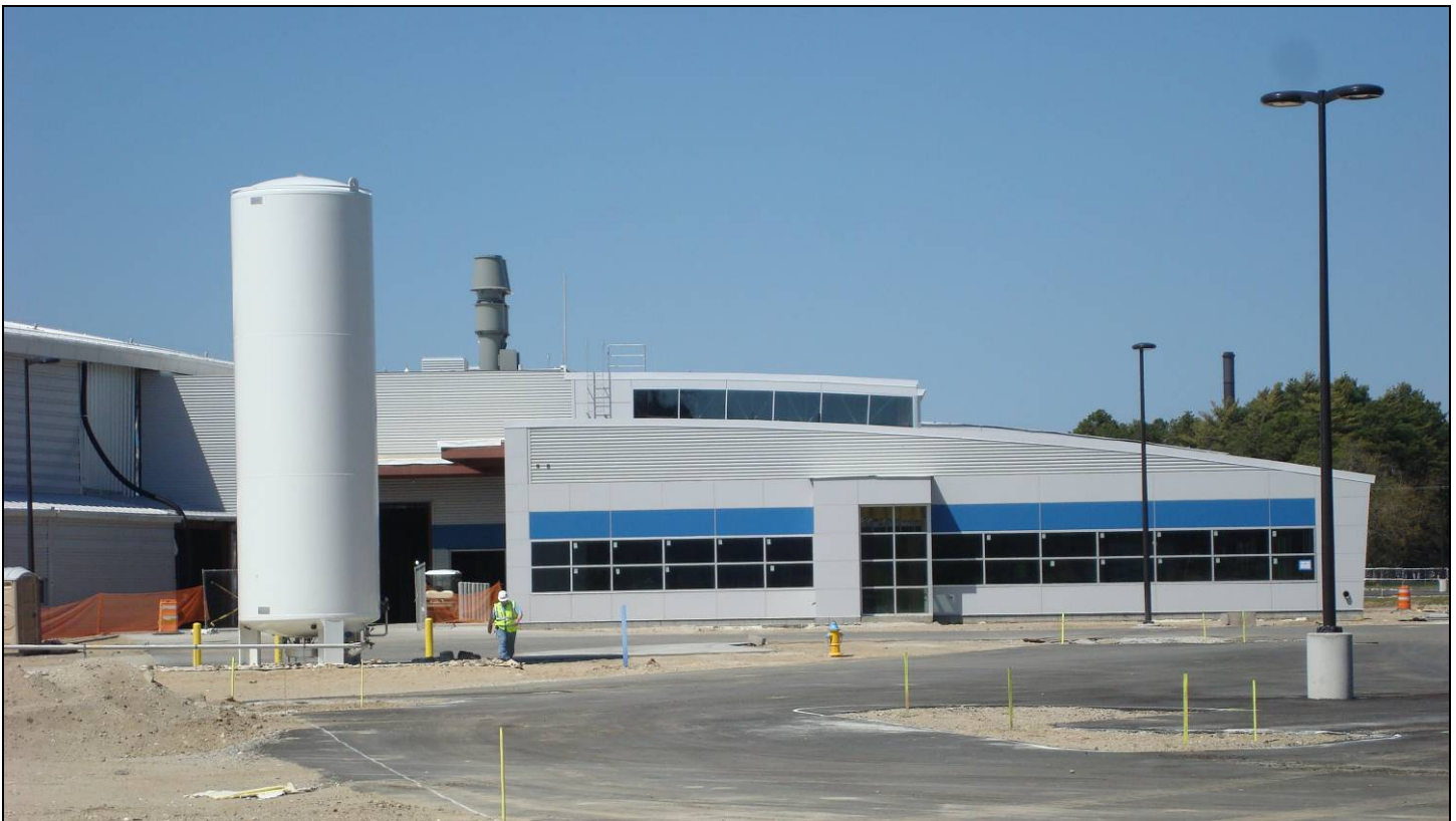
Figure 7. LOB 2 exterior siding nearing completion.
