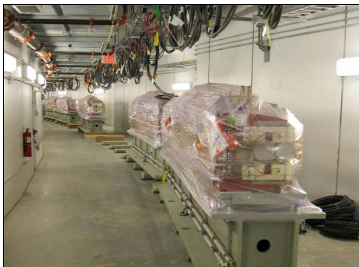
Figure 3. Girders in SR tunnel, pentant 1.
