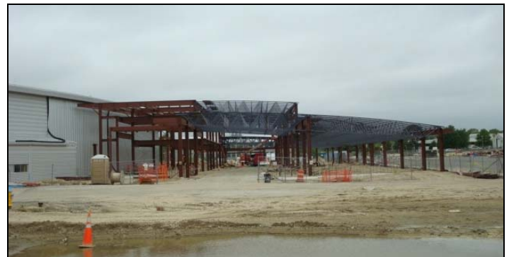
Figure 8. Structural steel provides the skeleton for LOB 1.
