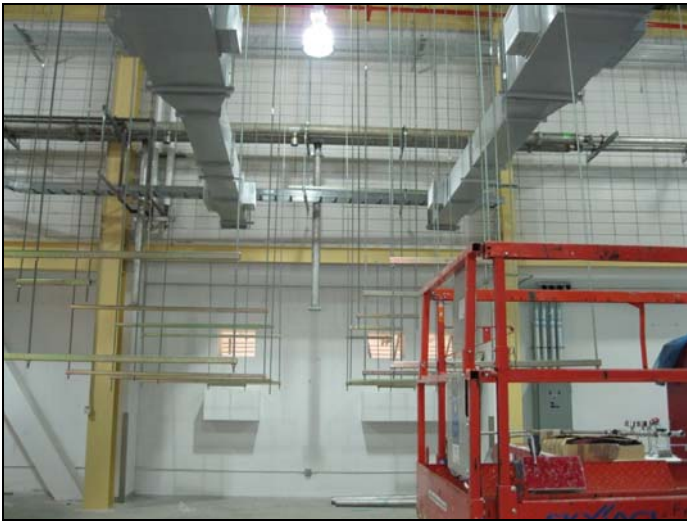
Figure 7. Preparation for transmitter installation in the RF building.
