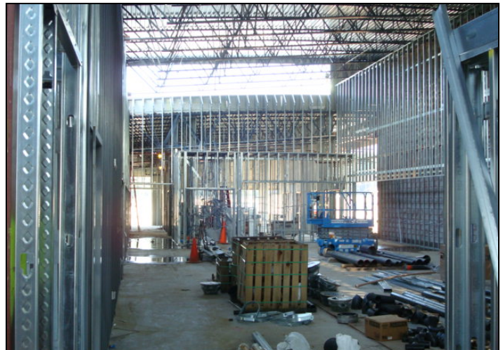
Figure 12. Partition walls in LOB 1 being studded out.
