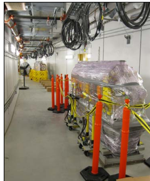
Figure 6. Second girder installed.
