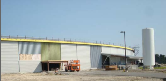
Figure 13. Pentant 5 ready for the final sections of ring building siding.
