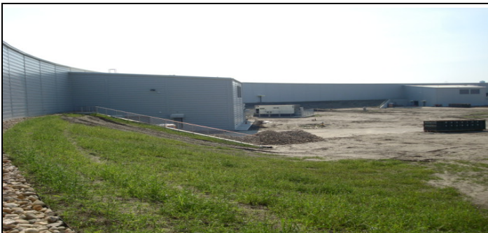
Figure 14. Grading of the interior courtyard is nearly complete.
