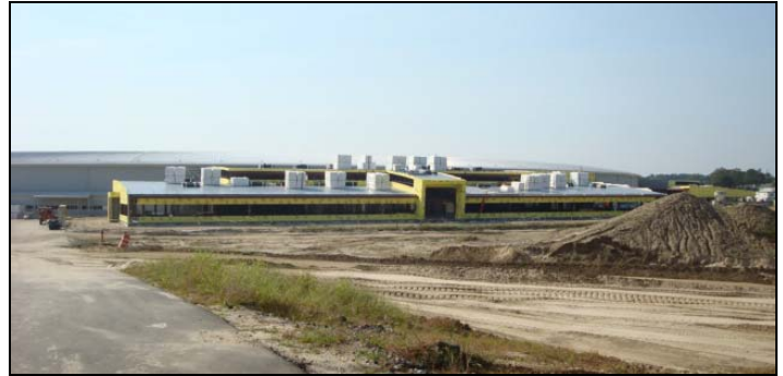
Figure 11. Work on the building envelope for LOB 2 progressed well in August.
