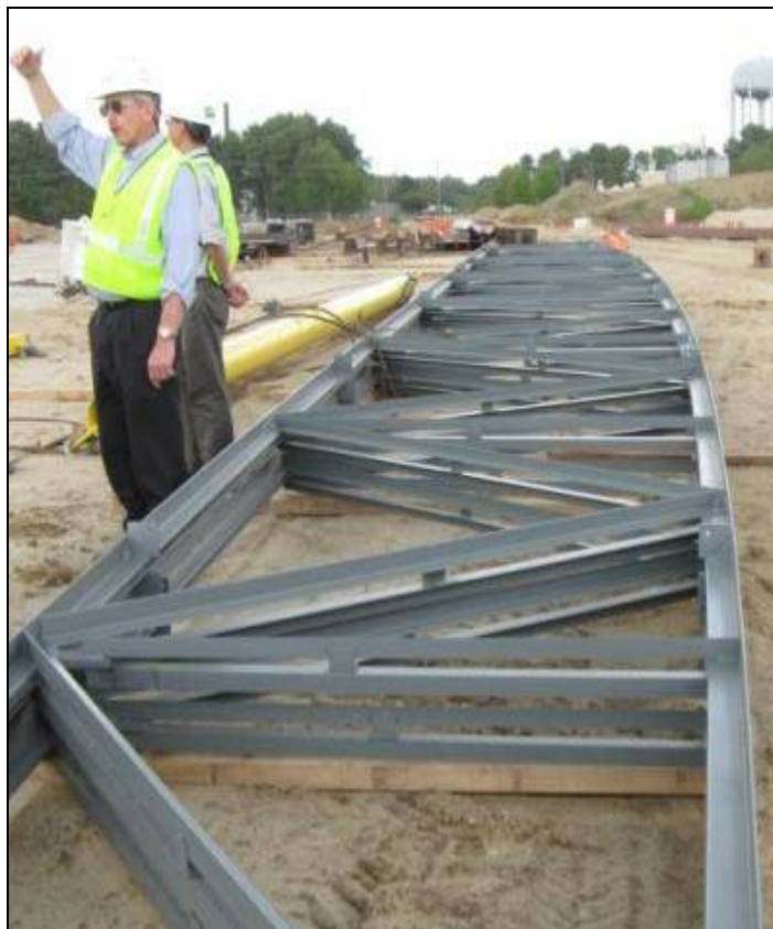
Figure 6. Curved roof joists for the Ring Building.
