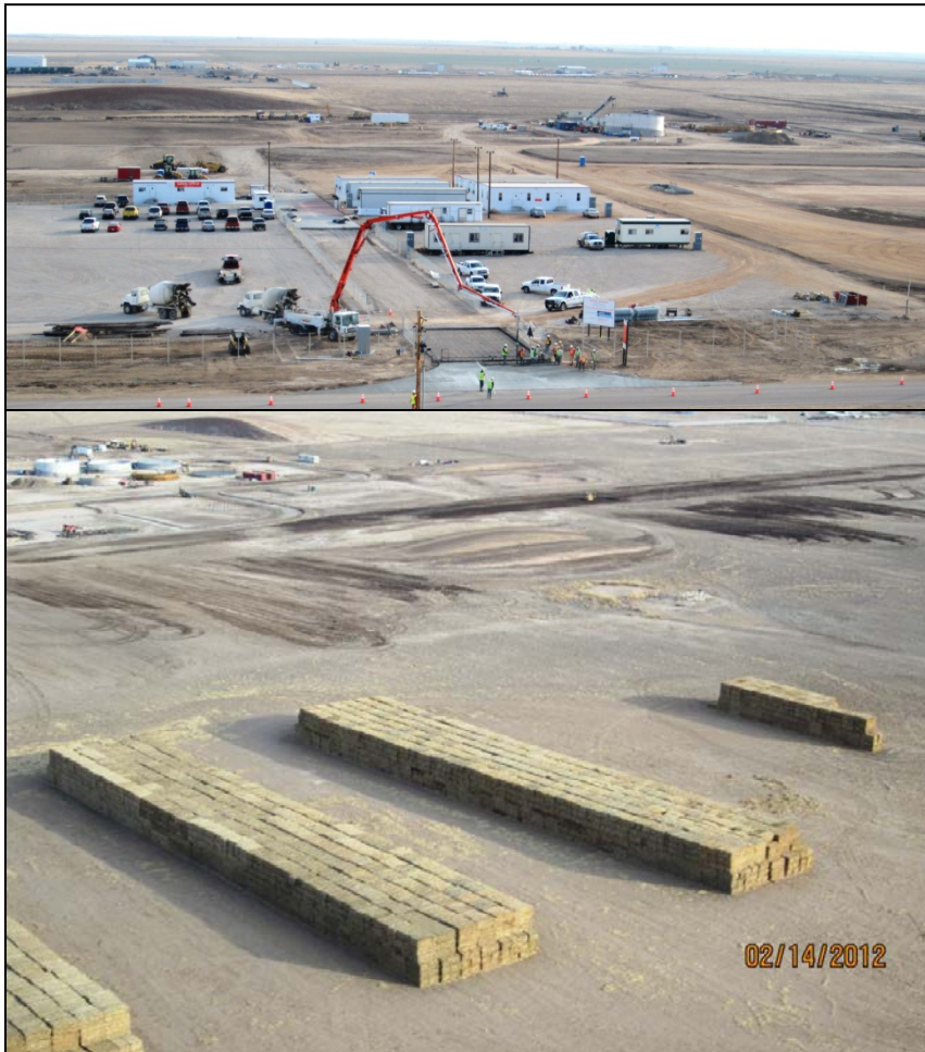
Figure 1: Abengoa biorefinery project stack yard.
