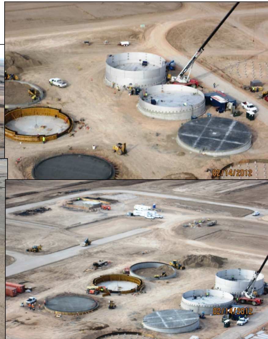
Figure 2: Abengoa biorefinery construction progress, Feb. 2012.
