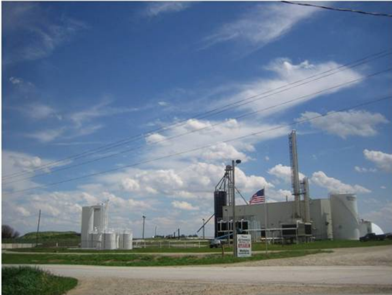
Figure 2: Fibright biorefinery undergoing renovation to cellulosic ethanol.
