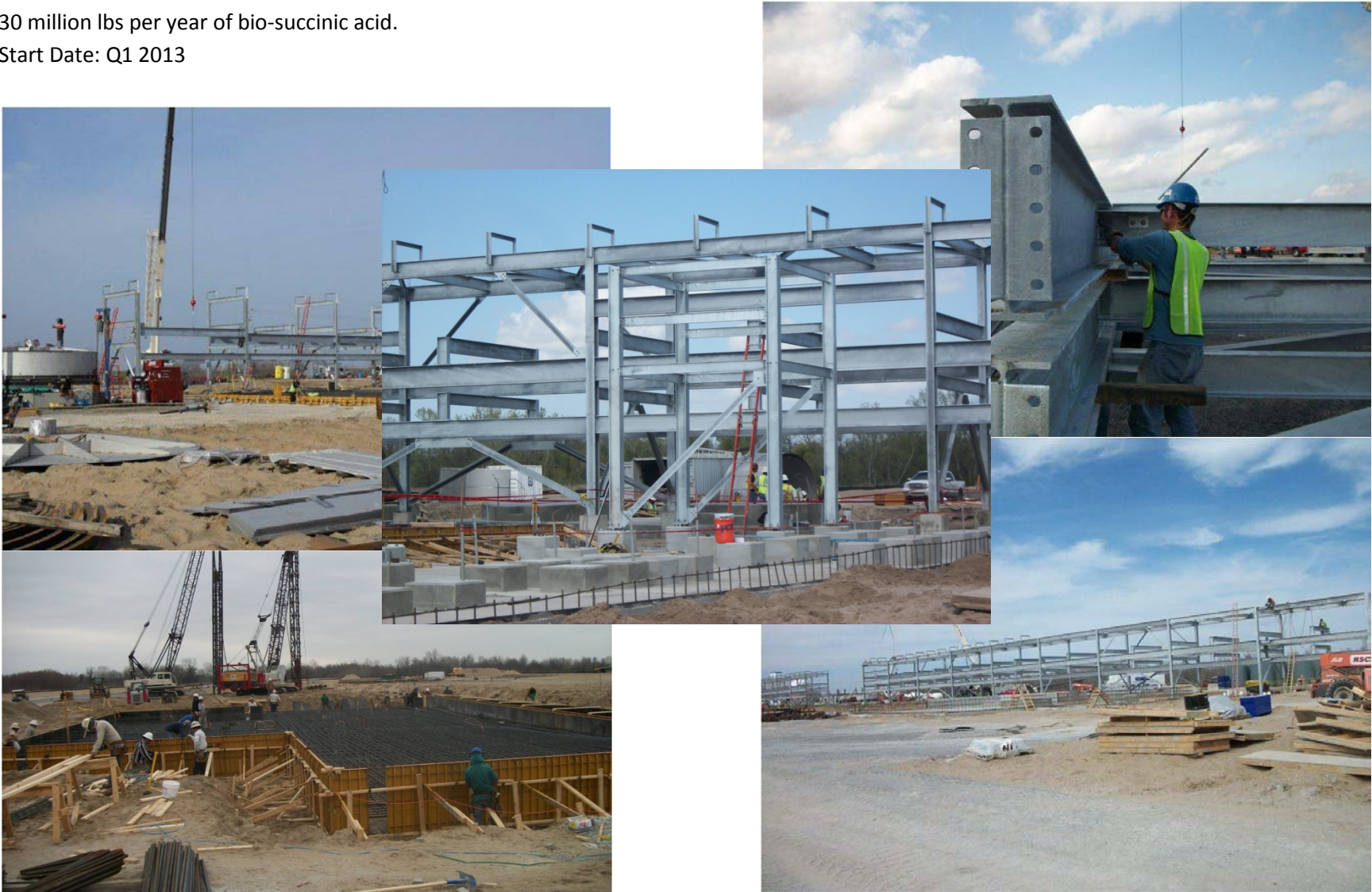
Figure 6: Myriant construction progress March 2012.
