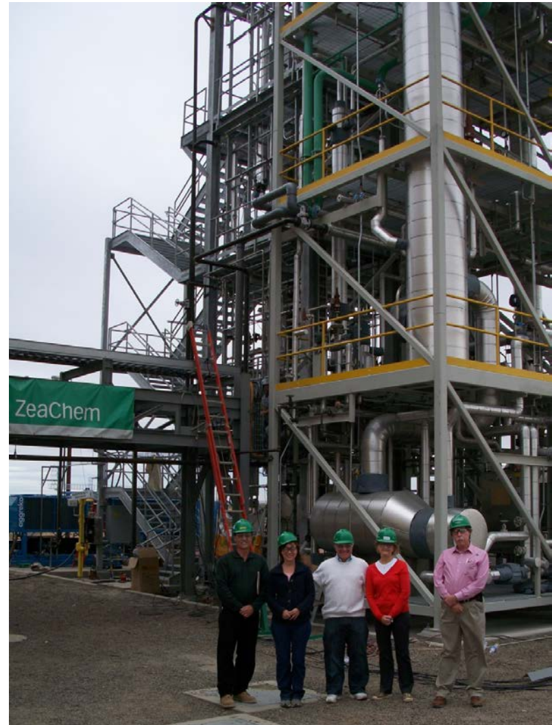
Figure 14: ZeaChem demonstration facility under construction, September 2011.
