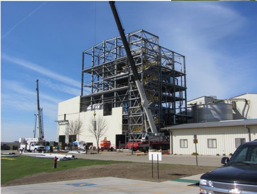
Figure 3: Gevo biorefinery undergoing renovation for biobutanol production.
