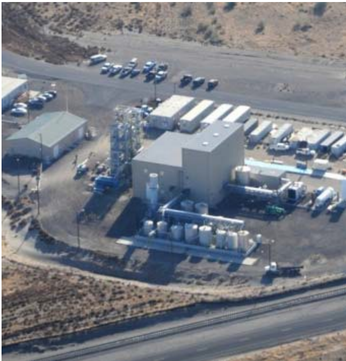
Figure 12: ZeaChem demonstration biorefinery, aerial view.
