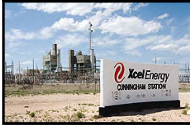
Figure 3- 5 Power Plant Located Across Highway NM 483 from IIFP Facility
