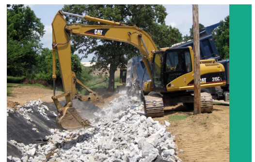
A contractor completes work on a streambank stabilization project in Lynn, Ark.
