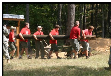
Youth volunteers carry materials to the bridge construction area.
