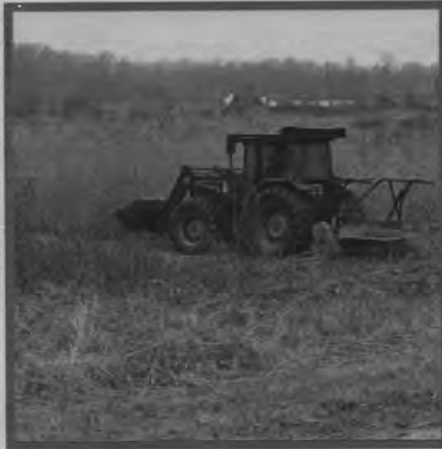
Clearing the site of all standing vegetation
