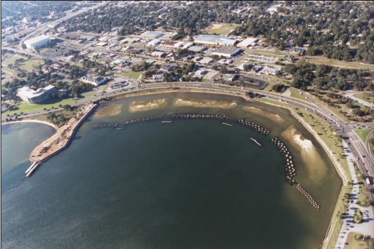
Figure 3: Aerial View of Project Greenshores
