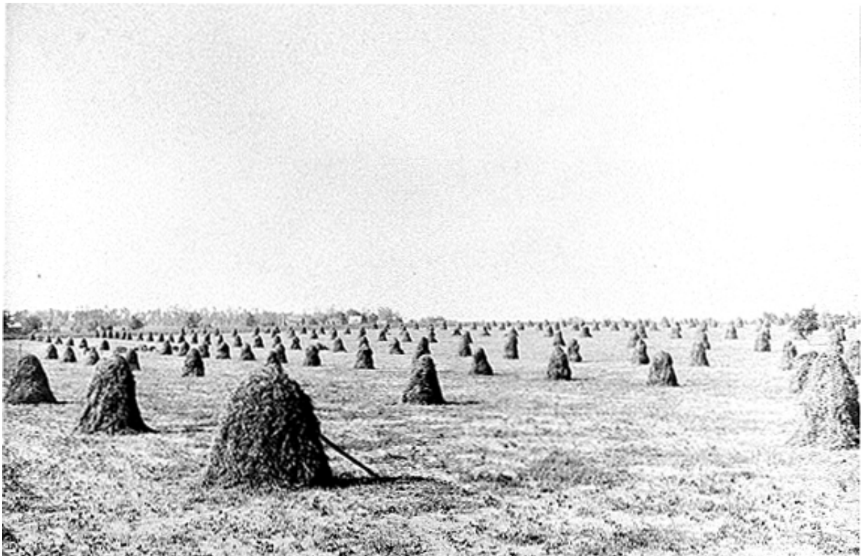
Figure 10. Agricultural land on Lowndes County around the turn of the century. Wooded land on the distant left is probably wetland, unsuitable for farming. The long vista in center where no tree line is visible indicates the vast extent of conversion of former longleaf pine lands to agriculture.
