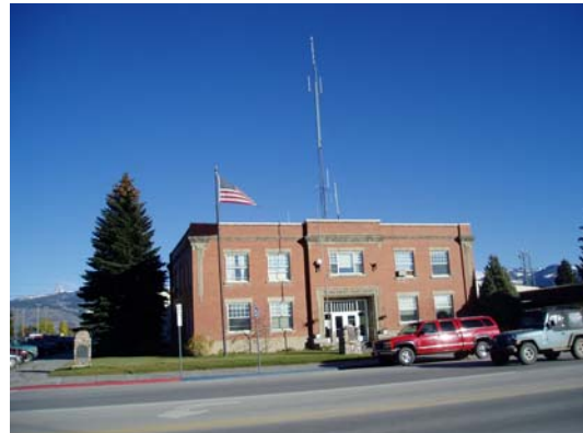
Figure 2: Teton County Court House in Driggs
