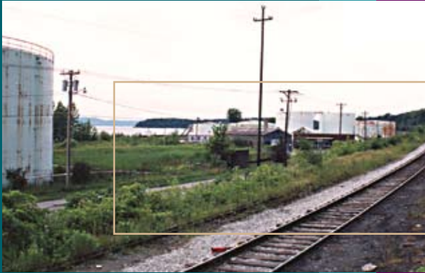
Prior to redevelopment, the banks of Lake Champlain were dotted with old oil tanks.
