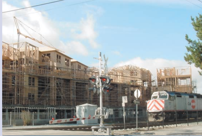
Construction underway on Phase I of the Franklin Street project, which will provide 206 residential units at the Redwood City Caltrain Station.
