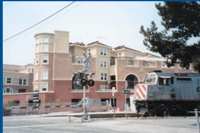
Phase I of the Franklin Street Project, near completion. The project received $1.2 million in TOD Incentive Program funds.
