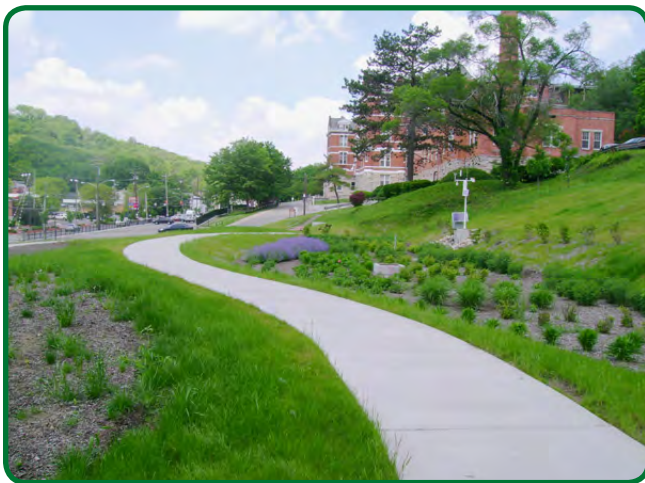
Rain gardens at the HUD-owned St. Francis Senior Apartments replaced excess pavement to reduce stormwater runoff. A monitoring station, pictured at right, measures runoff levels. Photo courtesy of EPA.
