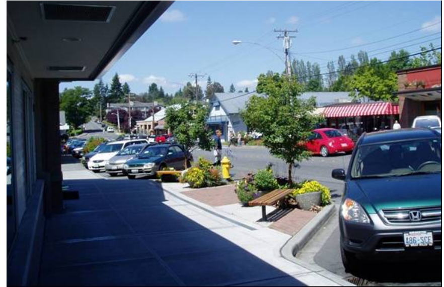
Figure 38: Mid-block curb extensions, Bainbridge Island, WA
