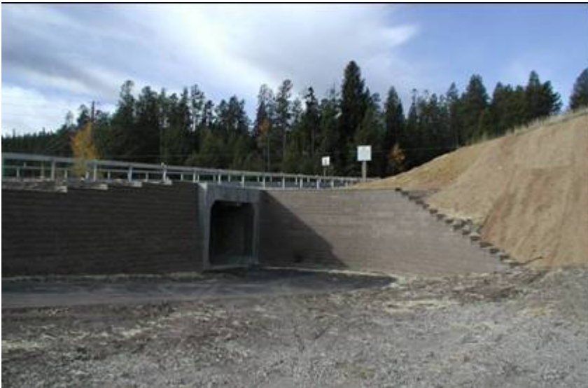
Figure 41: Grade separated crossing, Wilson, WY
