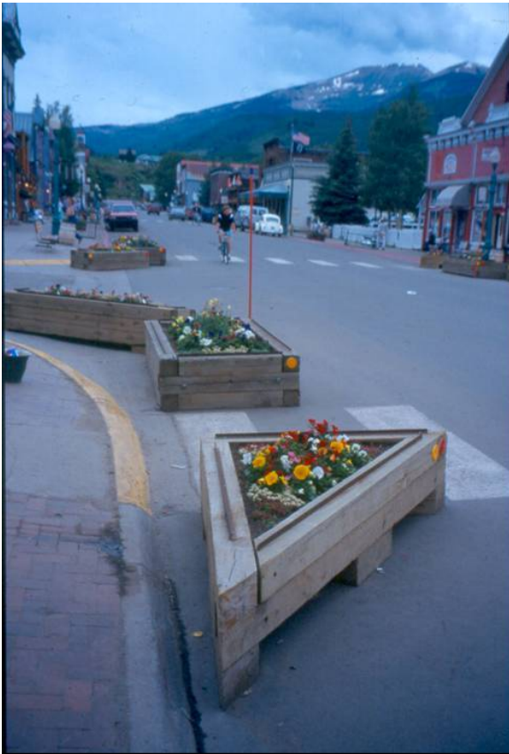
Figure 42: Temporary (summer) curb extensions, Crested Butte
