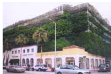
A variety of techniques can be used to improve the aesthetics of parking structures. Surprisingly, all of these images are parking garages.
