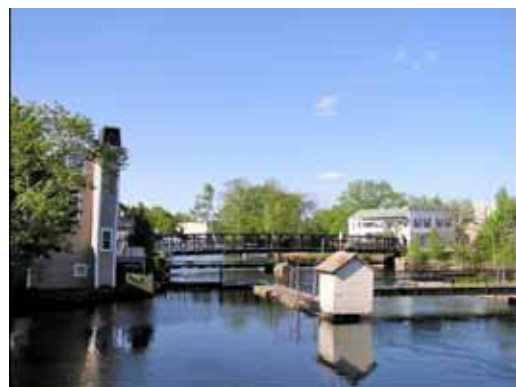
The Gold Street footbridge in Lakeport will be used by the W.O.W. bike trail to cross the Winnepesaukee River just to the east of Elm Street Bridge.
