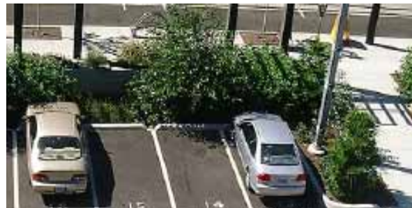
These parking lot basins capture stormwater runoff. Note the gap between spaces that allows water to flow into the basin.
