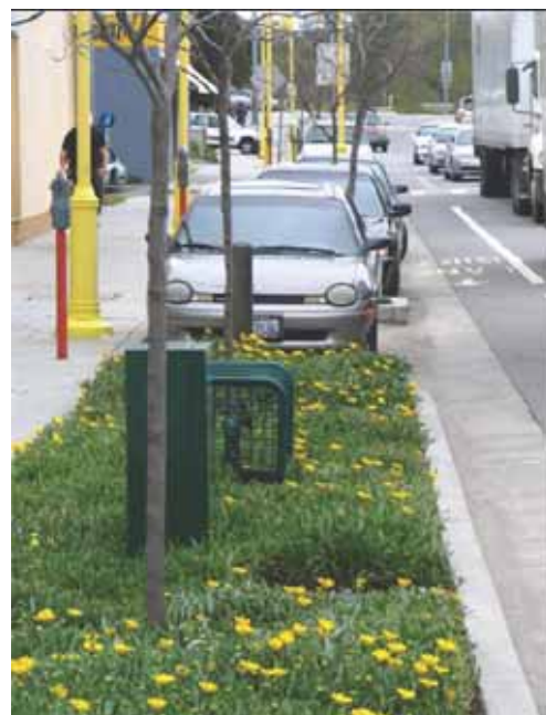
Street features such as this planting strip can add aesthetic appeal while absorbing stormwater runoff.
