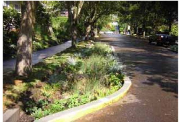
On this street, curb extensions capture stormwater.
