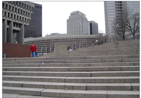
Fig. 18 A view from Congress Street looking west toward the main plaza space and 123 Center Plaza.
