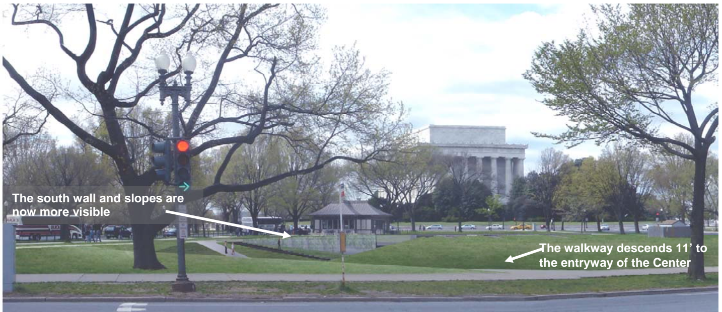
Revised June 2009 submission: View from corner of 23 rd Street and Constitution Ave The exhibit skylights are less visible because the grade of the site has been raised and the skylights are now flush with the grass. The south wall of the building and the walkway and adjacent slopes are now more visible.
