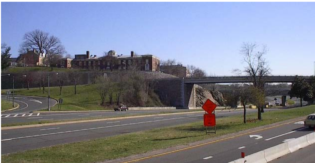
Old Naval Observatory overlooking Center Project Sector
