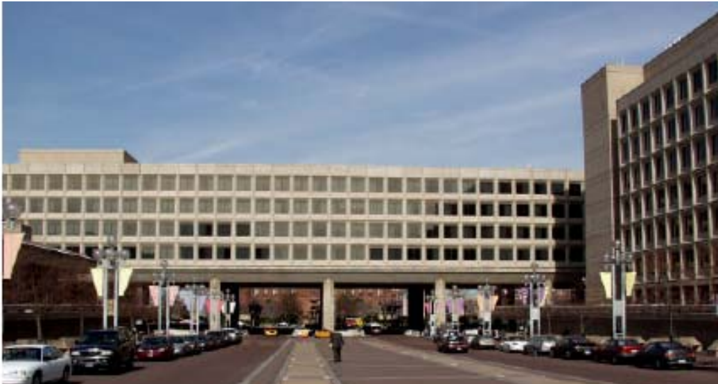
AXIAL VIEW OF 10 TH STREET PROMENADE LOOKING NORTH BENEATH FORRESTAL BUILDING
