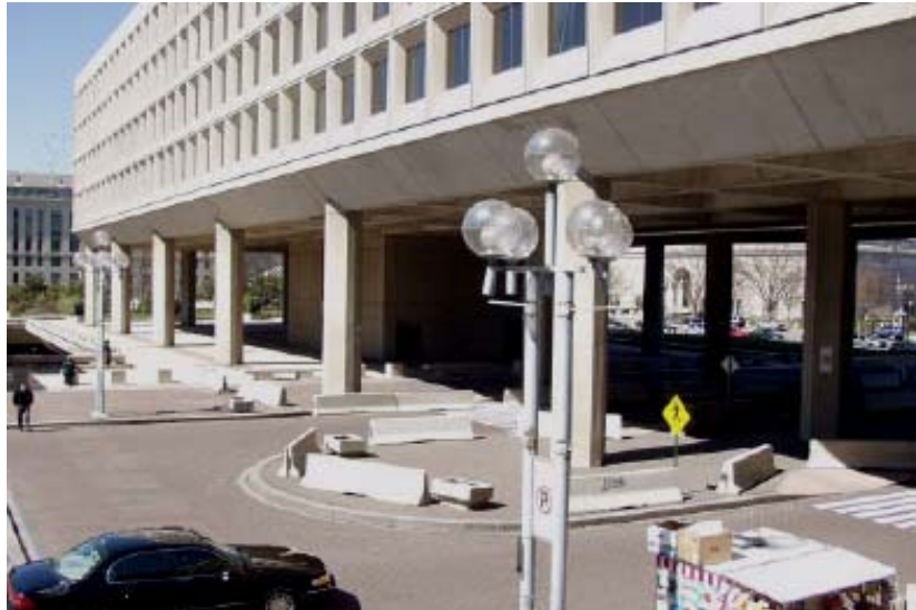
EXISTING TEMPORARY VEHICLE BARRIERS BENEATH BUILDING
