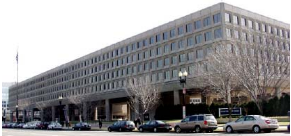
FORRESTAL BUILDING AS VIEWED ALONG INDEPENDENCE AVENUE, SW
