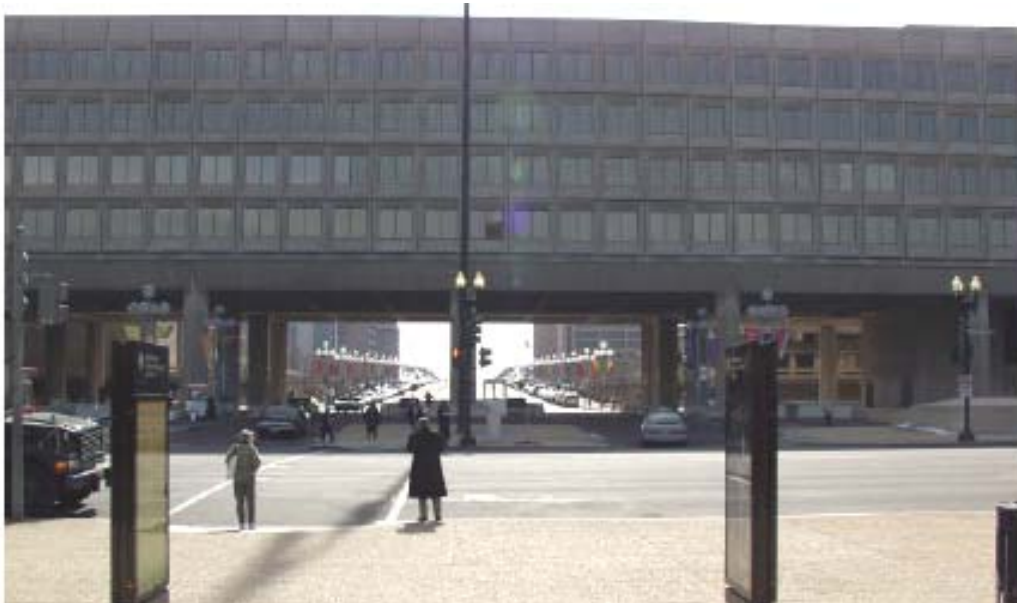
AXIAL VIEW OF 10 TH STREET PROMENADE LOOKING SOUTH BENEATH FORRESTAL BUILDING
