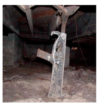
"I found a tire jack being used for structural support in a crawlspace"
