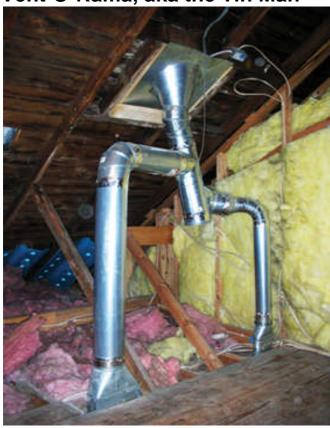
"The attic space was the full service venting location. The right-side venting came up from the water heater in the basement. The larger vent on the left arrived from the microwave exhaust fan in the kitchen and they all were heading out the roof through a non-functioning powered attic fan."
