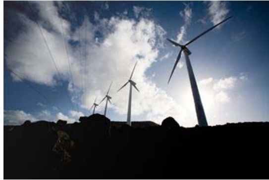
Four 225-kilowatt wind turbines help produce power for Ascension Auxiliary Airfield, a small base belonging to the 45th Space Wing. The base is located on the British-owned island of Ascension, which is positioned in the South Atlantic Ocean several thousand miles from the coast of Africa. (U.S. Air Force photo/Lance Cheung)
