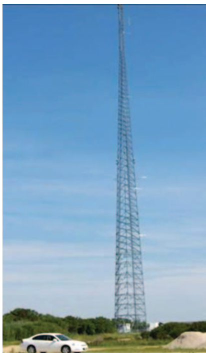
As part of a wind resource assessment effort with the U.S. Coast Guard, NREL provided Cape May (in New Jersey) with anemometers and wind vanes installed at 30, 44, 74 and 97 meters on an existing 109-m tower. Credit: Richard Ker, PIX 15661.
