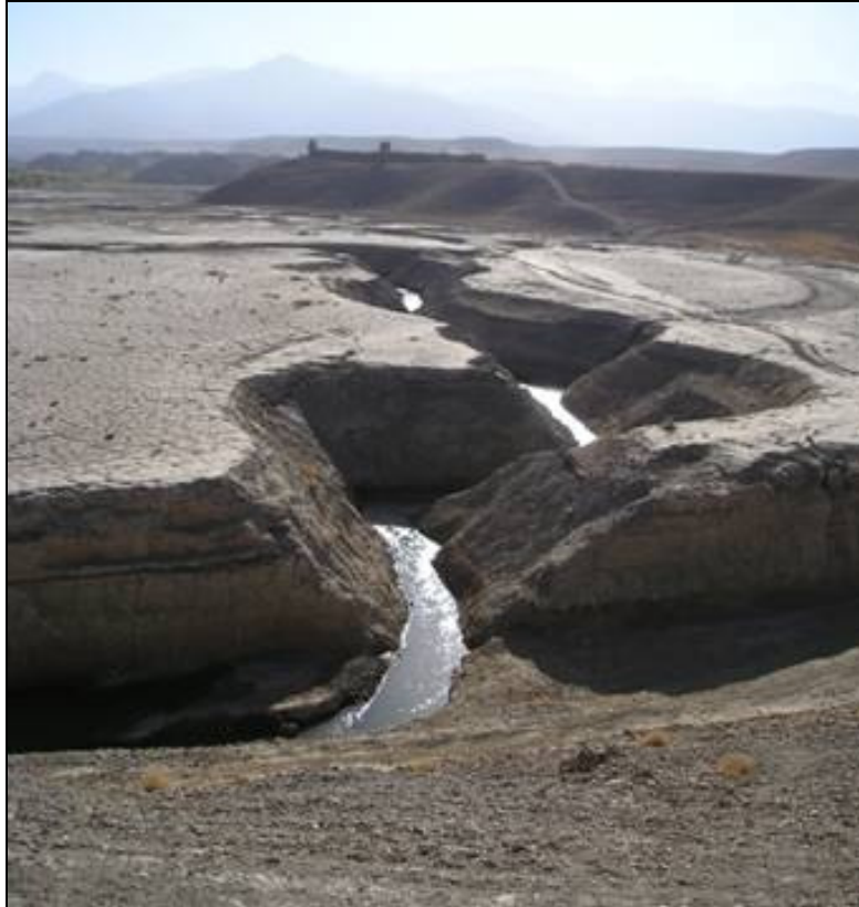
Figure 7-1 – Surkhab Dam, Logar, View from Top of Dam Downstream at Reservoir
