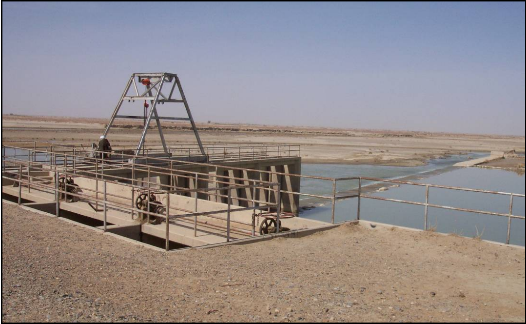
Figure 4-5 – Concrete Irrigation Diversion with Sluice Gates (Darweshan, Helmand Valley)
