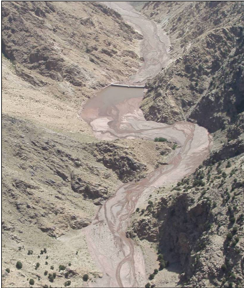
Figure 4-20 – Upstream of the Filled Reservoir (Oosterkamp, 2009)
