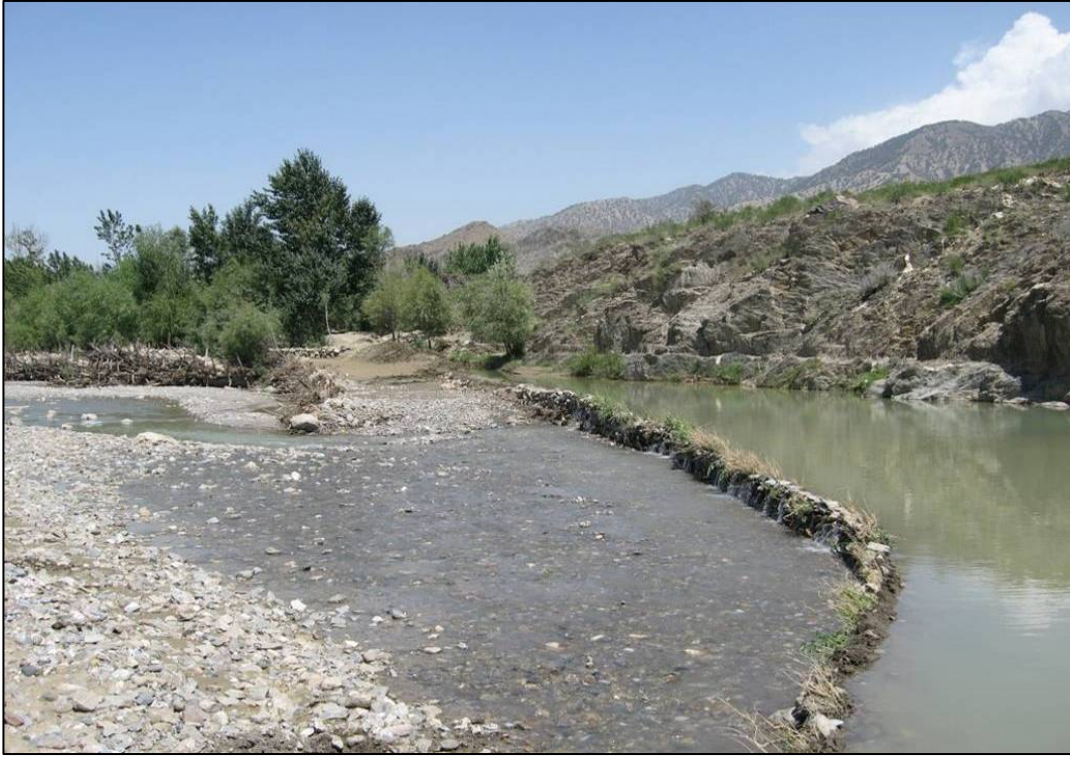
Figure 4-4 – Traditional Irrigation Diversion Structure (Bermel Valley, Paktika)
