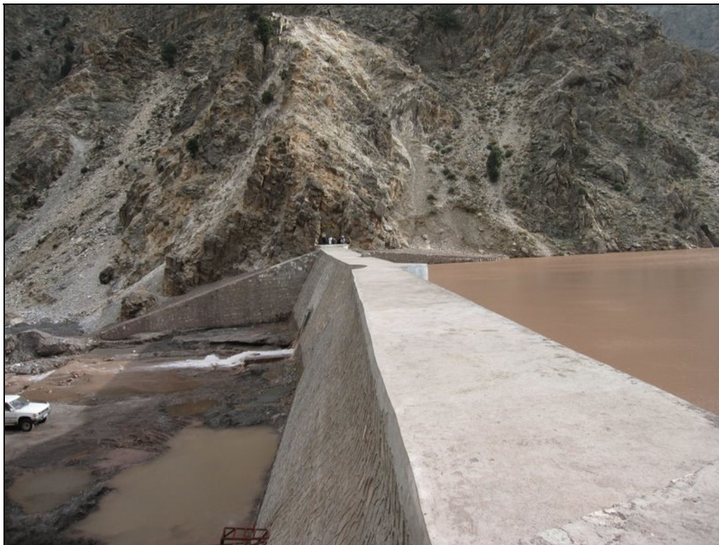
Figure 7-2 – Hezarak Dam, Nangarhar View along Top of Dam (Oosterkamp, 2009)
