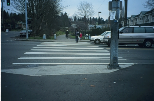
Figure 8-11. Continental crosswalks combined with alternative measures, such as pedestrian actuated traffic controls, enhance pedestrian crossing.
