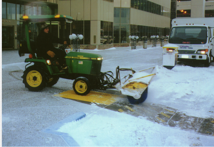
Figure 6-6. A snowplow with a brush that is used to remove snow from sidewalks in Anchorage effectively removes snow from truncated dome surfaces.
