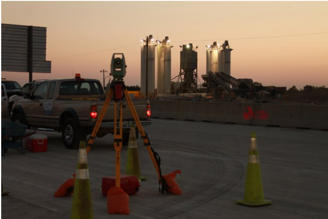
Figure 2. Total Station at PCC Paving Site.
