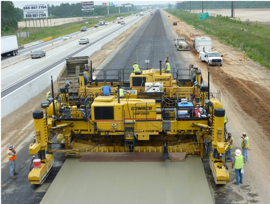
Figure 4. Stringless PCC Paving.
