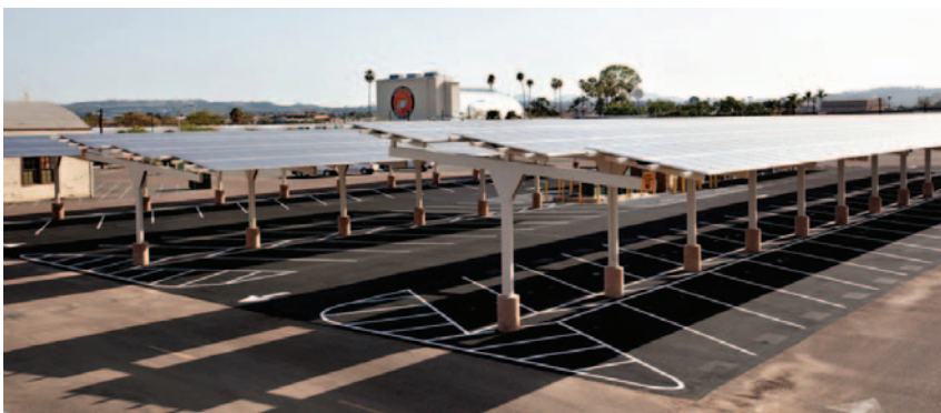
As part of its move toward net zero energy, MCAS Miramar installed this 250-kilowatt solar carport in April 2010. Courtesy of MCAS Miramar
