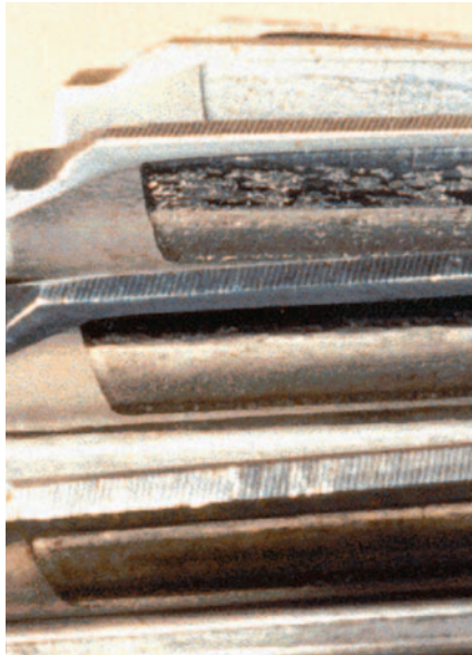
Tests conducted at the NWTC look at ways to arrest micropitting (flaking of surface layers) on wind turbine gear that can lead to serious operational problems. PIX 09992
