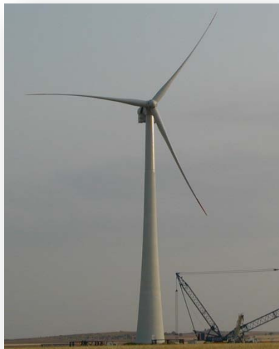
Innovative Tall Towers
