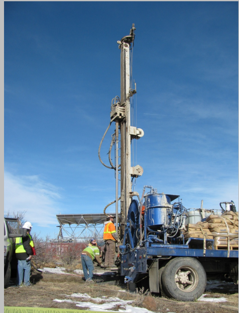
Drilling rig on South Table Mountain, testing for installation of geothermal heat pump showcase system at NREL.
