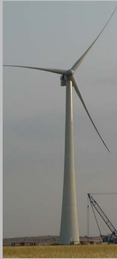
Innovative Tall Towers
