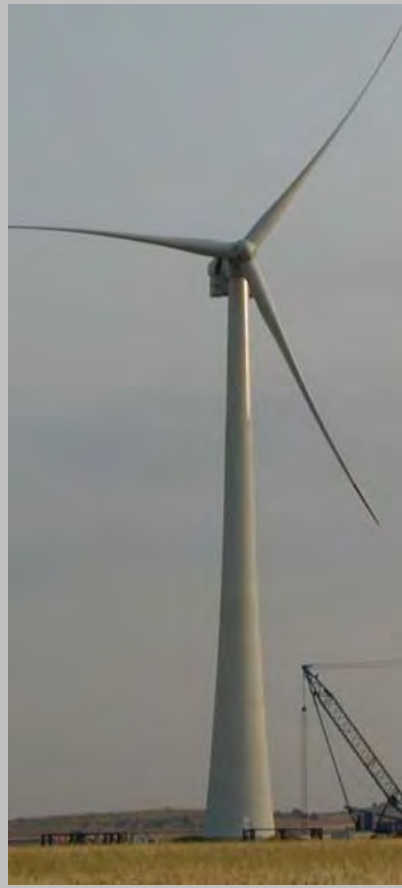
Innovative Tall Towers
