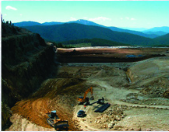
Workers in the foreground are preparing the Luttrell Abandoned Mine Waste Repository for 2003 remediation work. Previously placed abandoned mine wastes with temporary cover are shown in the background.
