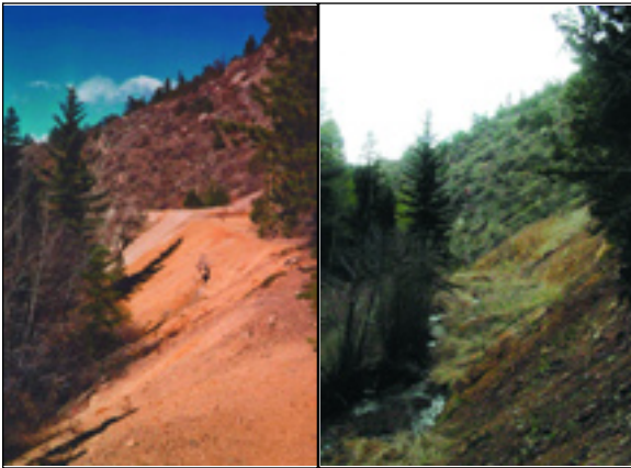
Little Bear Abandoned Mine Site, Arapaho National Forest, south of Idaho Springs, CO. Sulphide-bearing waste rock pile, discharging directly into Little Bear Creek, is stabilized and vegetated to stop sediment and heavy metal runoff. Such clean up efforts can be complicated, time-consuming, and expensive.
