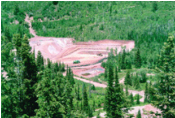
The excavated repository at American Fork before material placement.
