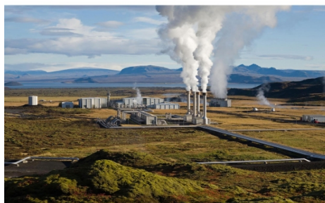
Germencik Geothermal Power Plant
