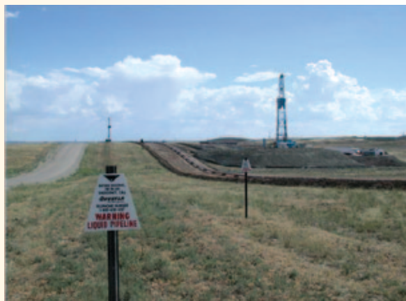
Bury gathering lines adjacent to the road
