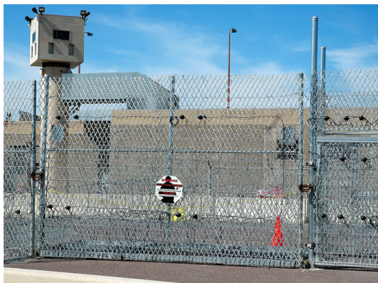
Security barriers provide one of the many layers of physical protection.
