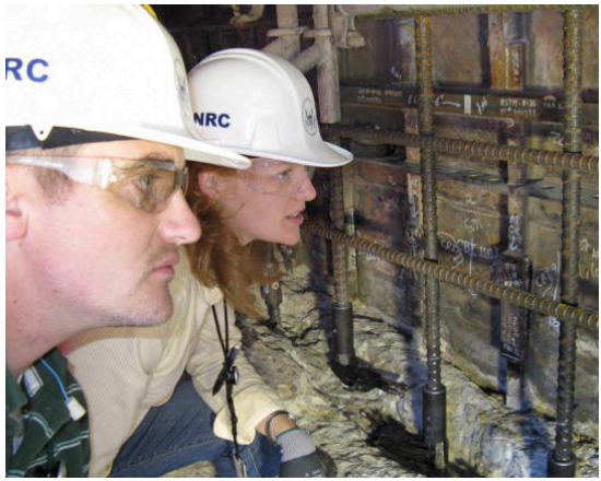
An NRC inspector gathers information at a nuclear power plant.
