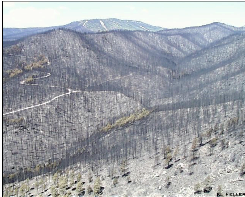
Pueblo Canyon west of Los Alamos town site following Cerro Grande Fire.
